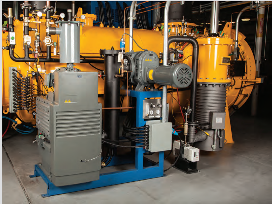
■ An example of a typical vacuum pumping system
