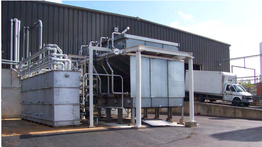
Figure 8 - Solar Atmospheres External Cooling Components
