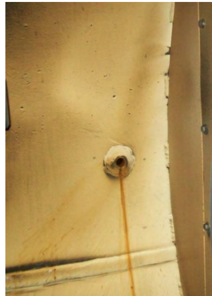
Figure 10 - Pipe Leakage Expanded From Figure 9
