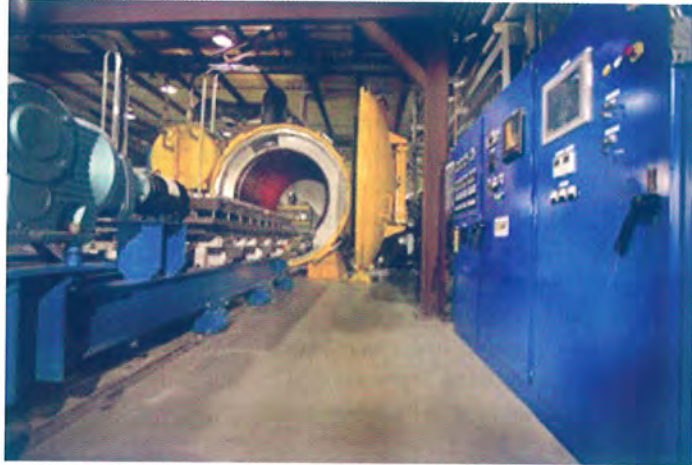
Fig. 4b. Car-bottom furnace for 10,000-pound loads
